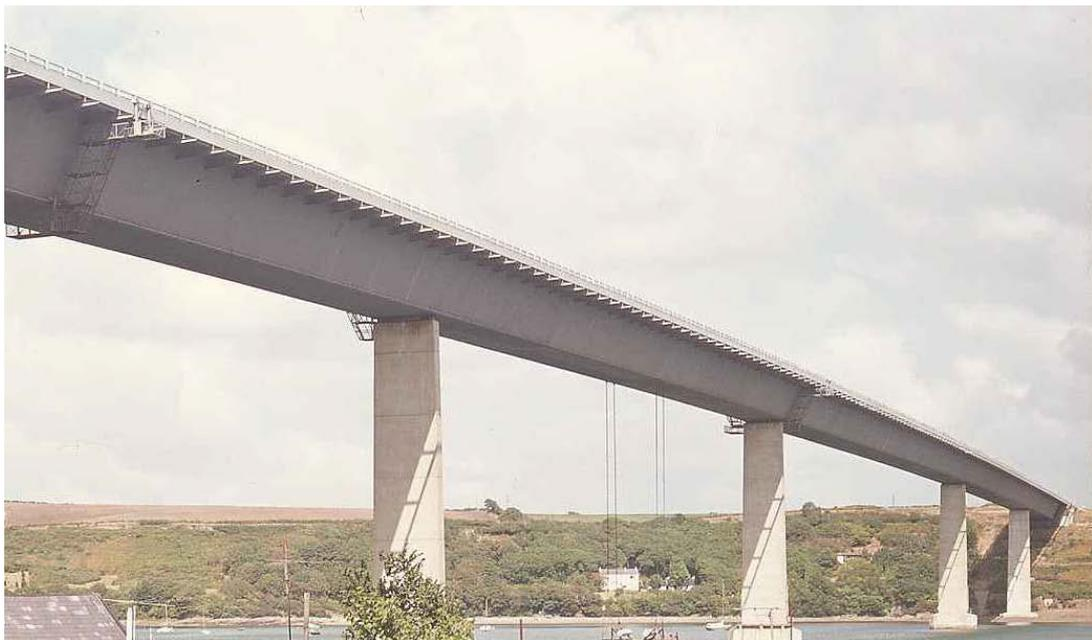
**Fig. 7.3 Box Girder Bridge Sections with One Box**
