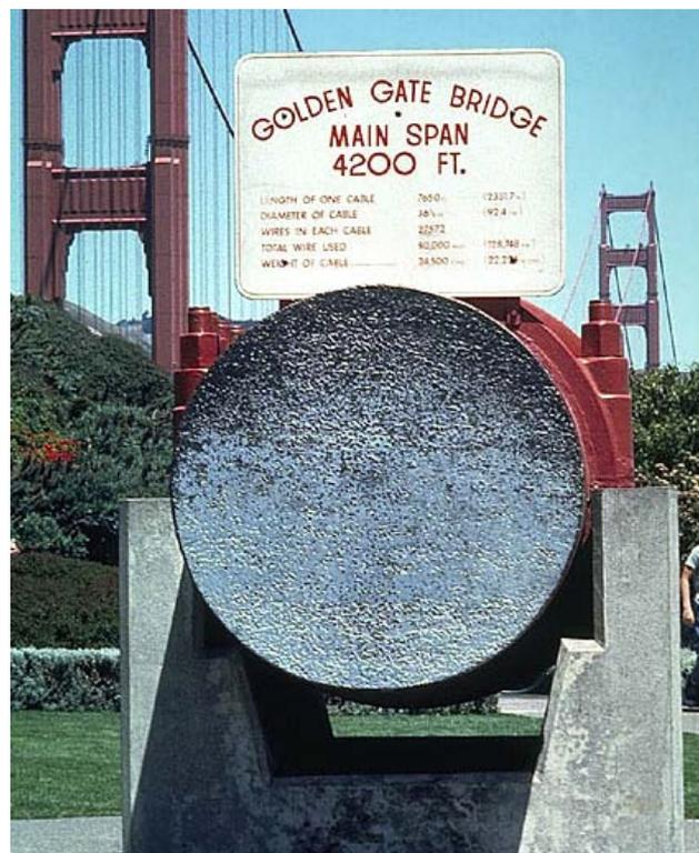
**Fig. 1.11b Section of a suspension bridge cable, showing it is made up of a bundle of small cables**
