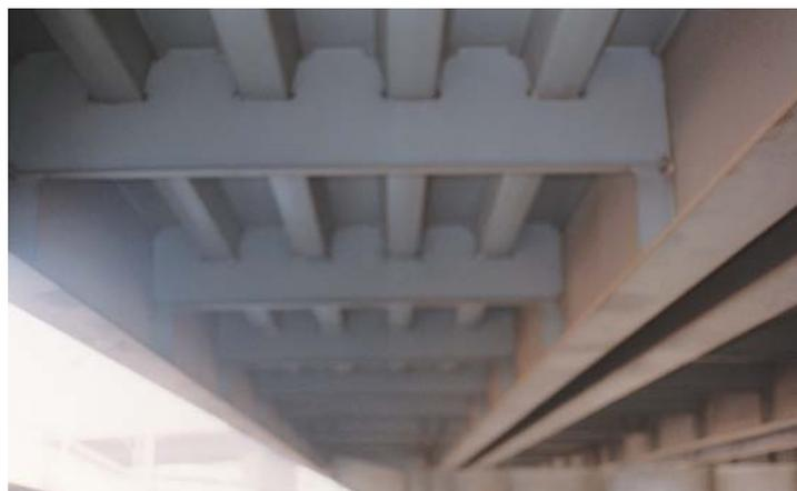
**Fig. 4.2 Roadway Bridge Floors: c) Orthotropic Plate Floors**
