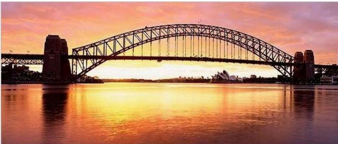
**b) Sydney Harbor Arch Bridge, completed 1932. Almost the longest arch bridge in the world (longest is Bayonne Bridge, New York, completed a few months earlier, 1.5 m longer). Two-hinge arch, span between abutments is 503 m to allow unobstructed passage for ships in Sydney Harbor. Contains 50,300 tons of steel (37,000 in the arch). The widest (49 m) bridge in the world.**
