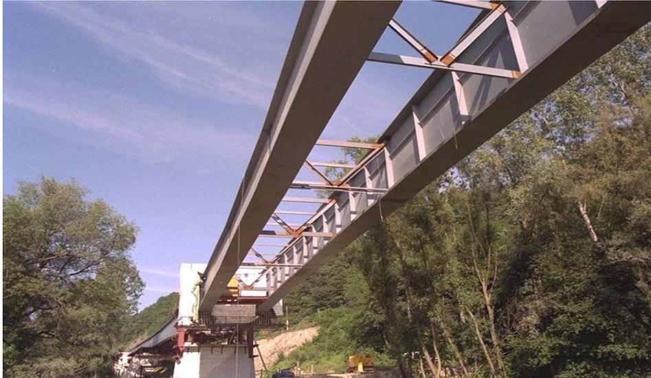
**Fig. 5.41 Cross Bracing for Deck Bridges - Intermediate Cross frames**
