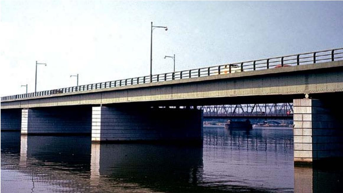
**(a) 14th Street Bridge over the Potomac River (USA). Continuous riveted steel girders. Note the absence of internal hinges, and the roller supports at the piers**
