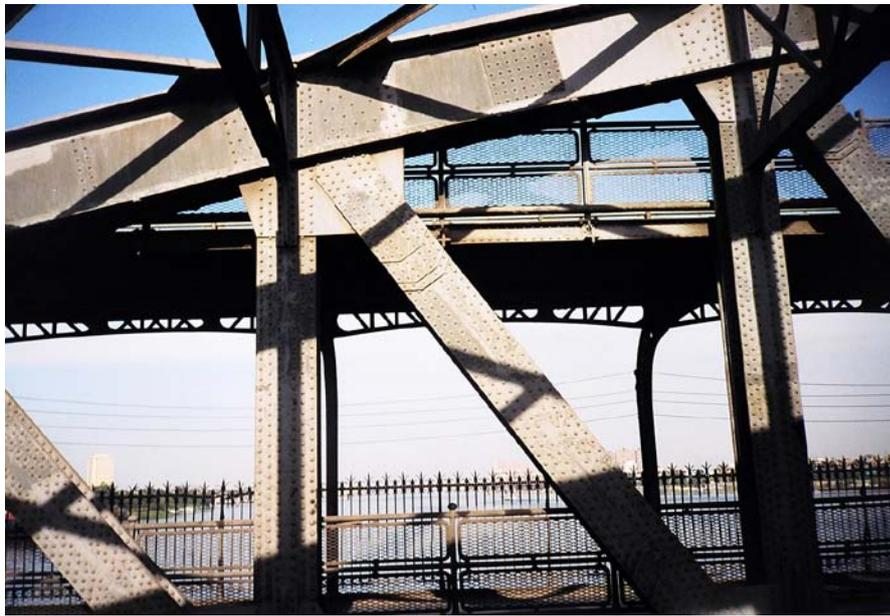
**Fig. 8.8 Bolted Truss Joints with Splice outside Joint**
