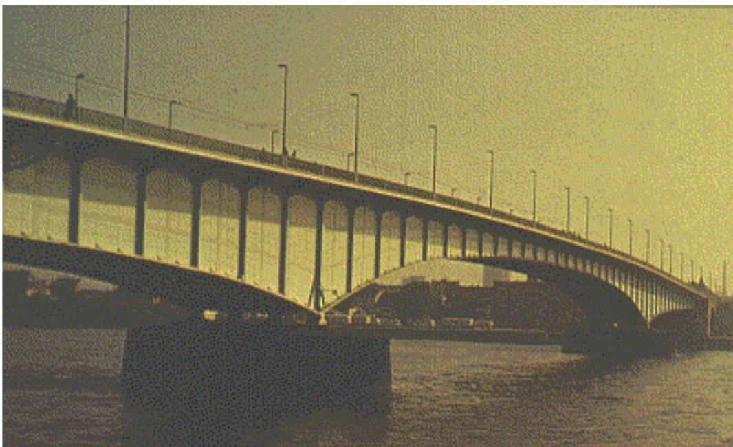
**Fig. 5.3 Plate Girder Bridge with Variable Depth**
