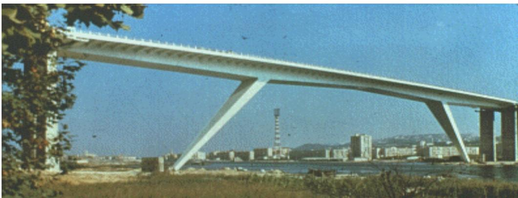
**Fig. 1.8 Bridge Systems Carrying Loads by Bending, Rigid Frames with Vertical or Inclined Legs**
