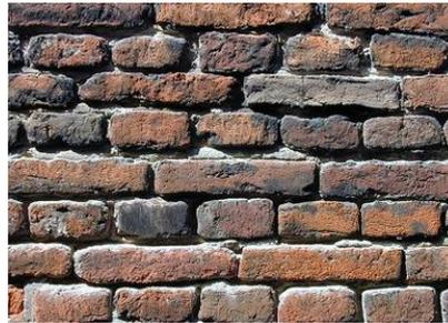
d. **Fourth class bricks:** These are over burnt bricks with irregular shape and dark colour. These bricks are used as aggregate for concrete in foundation, floors, roads, etc because of the fact that the over burnt bricks have compacted structure and hence, they are some times found stronger than even first class bricks.
