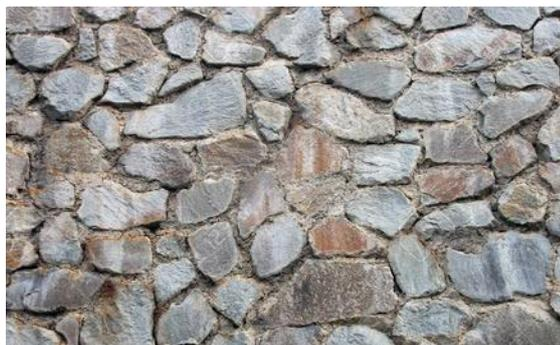
(i) **Uncoursed rubble masonry:** This is the cheapest, roughest and poorest form of stone masonry. The stones used in this type of masonry very much vary in their shape and size and are directly obtained from quarry. Uncoursed rubble masonry can be divided into the following.
