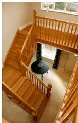
(iv) **Bifurcated stairs:** In this type of stairs, the flights are so arranged that there is a wide flight at the start which is divided into narrow flights at the mid-landing. The two narrow flights start from either side of the mid-building.
