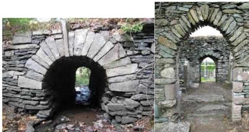
(ii) Brick arches: Can be constructed with ordinary or purposed made bricks. Ordinary bricks are not cut to shape of voussoirs & hence rough brick arches are formed. For getting the arch curve, joints are made wedge shaped with greater thickness at extrados and small thickness at intrados. Hence arch appearance is spoiled, thus rough brick arches are not suitable for exposed brick work. Purpose made bricks are special bricks of different sizes which are suitable for good quality arch work.
