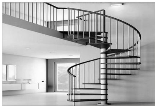
(vi) **Geometrical stairs:** This is similar to the open-newel stair with the difference that the open well between the forward and backward flight is curved. In this form of stairs, change of direction is obtained through winders.
