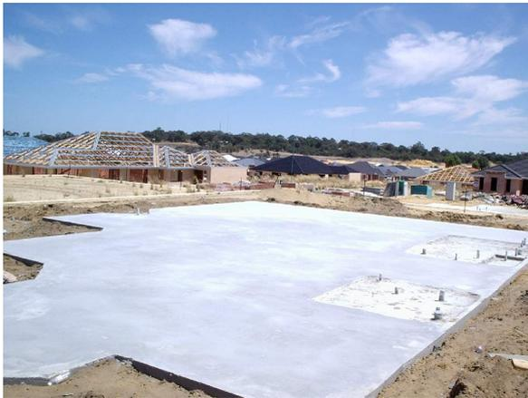
Figure 6.10: A slab foundation, built to spread the load of a smaller building.
