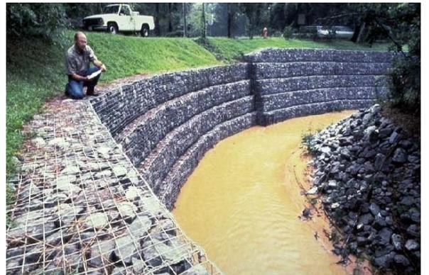
Figure 6.13: Stone-filled gabions, stabilising a river bank.
