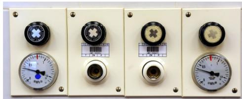
*Fig. 16-1 Central oxygen distribution panel
