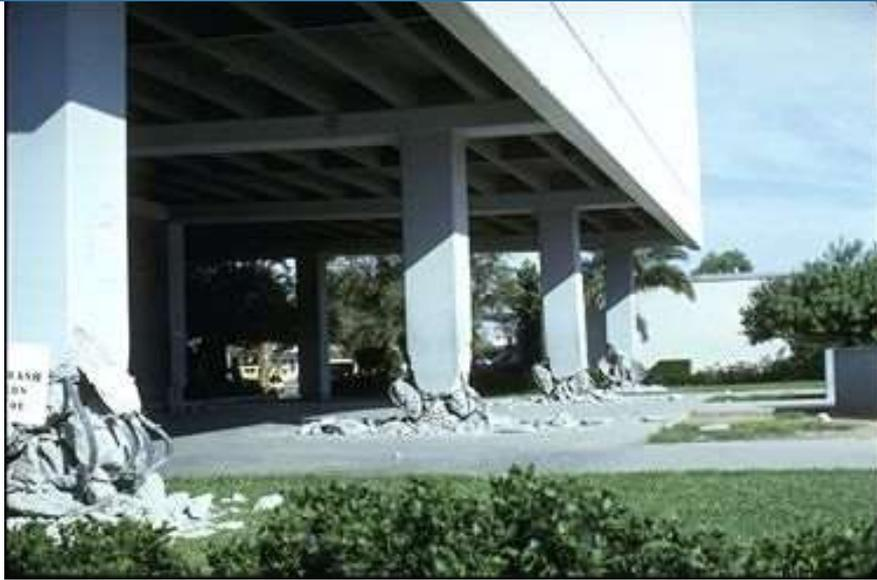
Crushing failure –
