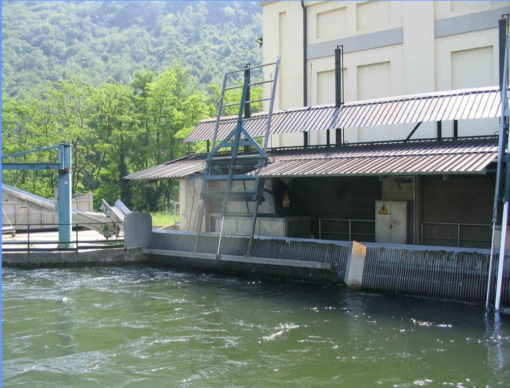
*The maximum possible spacing between the bars is generally specified by the turbine manufacturers. Typical values are 20-30 mm for Pelton turbines, 40-50 mm for Francis turbines and 80-100 mm for Kaplan turbines.*
