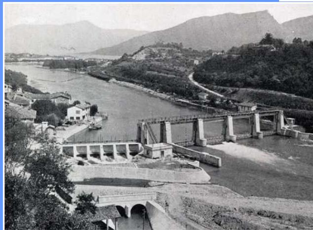
Gavardo: spillways with flat gates partly open to release ecological flow
