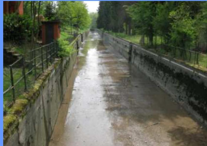
**5) channel for cobbles and gravel settling, looking downstream**
