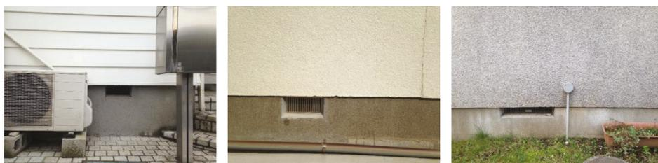
**Figure 2.** Underfloor openings for the natural ventilation in Tokyo, Japan.
